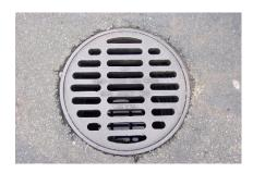
The City area storm drainage system consists of drains and underground pipes located in neighborhood streets, roads, and parking lots. Sewer pipelines carry household water to the Wastewater Treatment Plant, while water outside the home flow into a storm drain directly to a lake or river.
